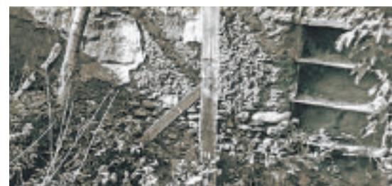
Shore-stones near the ground, earthen walls above
