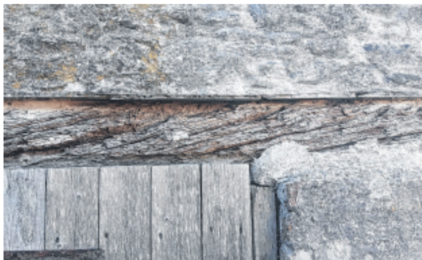
Ship's timber lintel in a shore-stone walled farm building
