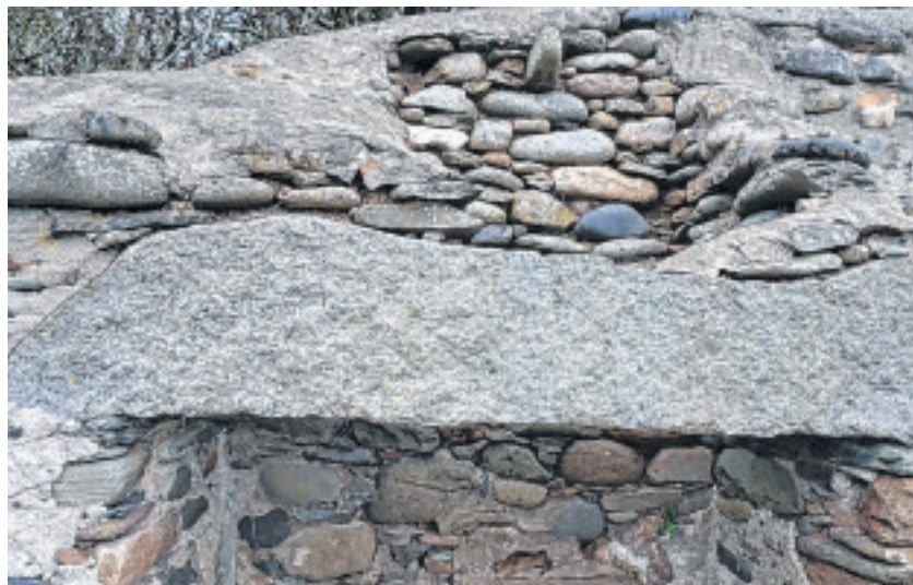
A near two metre long chiollagh lintel worked from a granite erratic boulder
