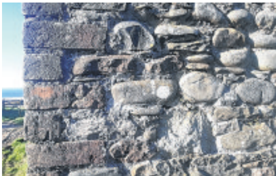
Shore-stone building walls with stone corners (left) and brick corners (right)
