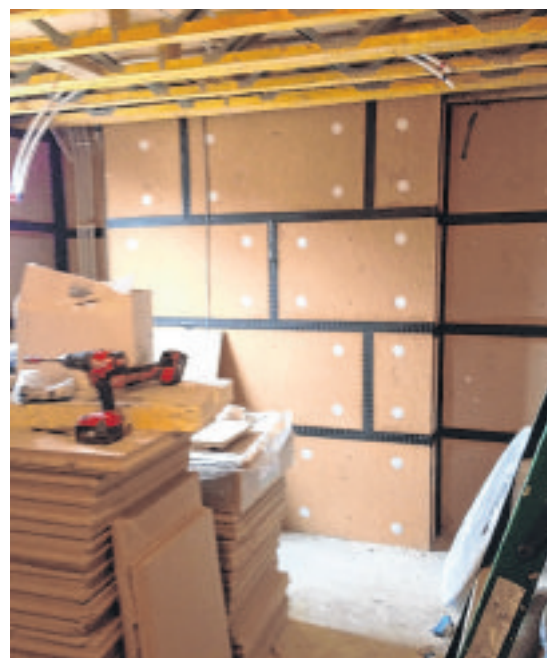
(Left) on the inside of the house, the external walls were given a coat of lime render before being lined with woodfibre insulation (right)
