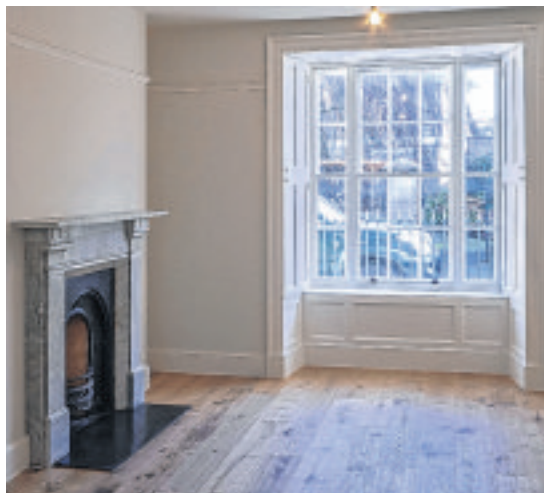
The replacement sash windows in the front rooms have slimline double-glazing units, while the timber panelling has been restored
