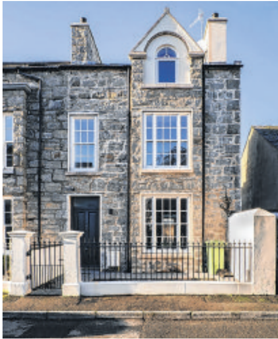
(Left image) The external walls were repointed using lime mortar, while modern materials complement the conservation area
