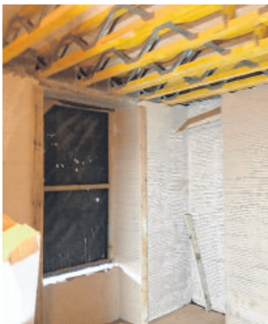
(Left) on the inside of the house, the external walls were given a coat of lime render before being lined with woodfibre insulation (right)
