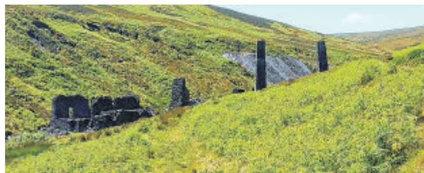
North Snaefell mine, aqueduct pillars carried water to the wheel
