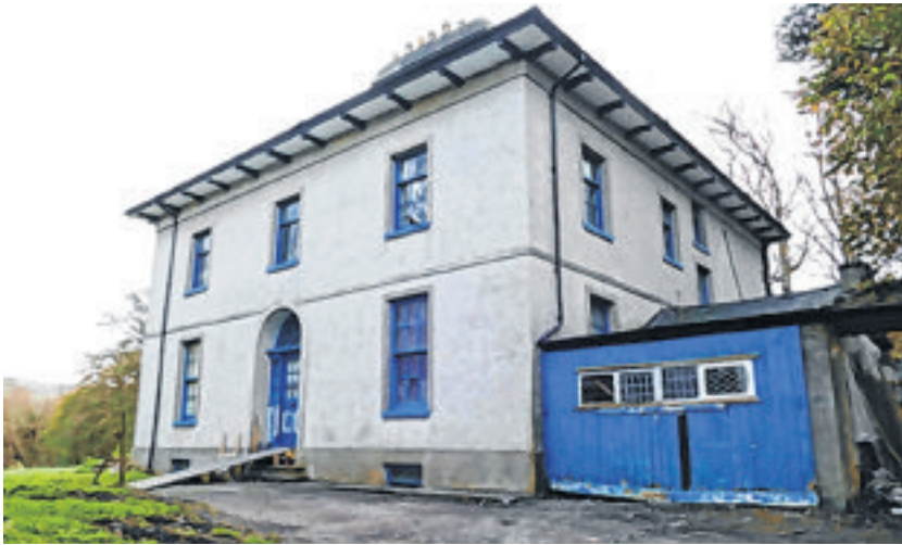
Glenfaba House which was demolished before any planning approval
