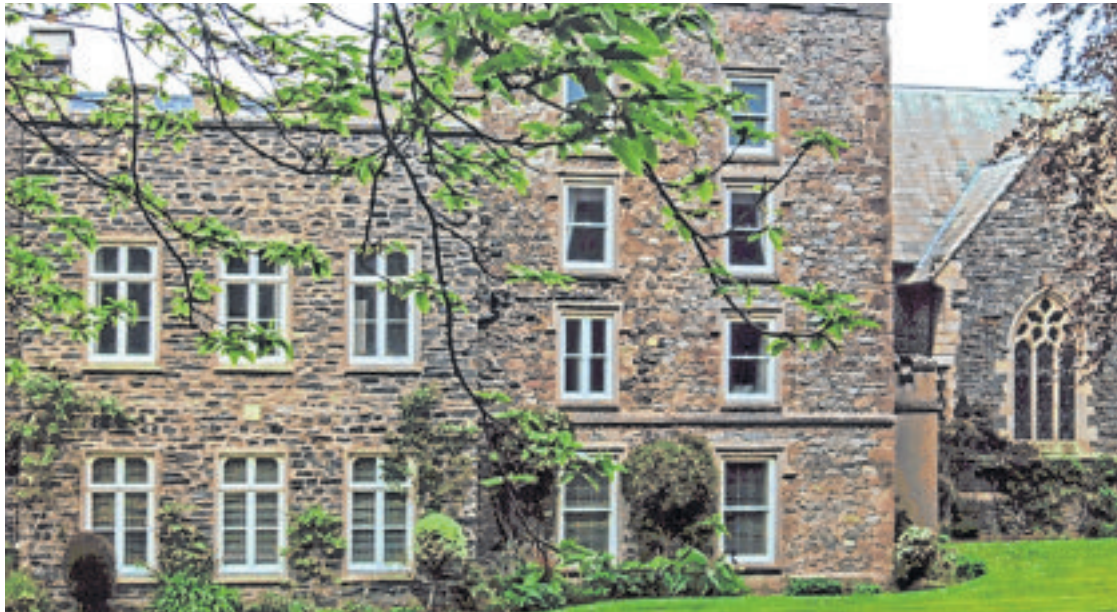
Bishops court Tower block with the Thomas Brine extension to the left
