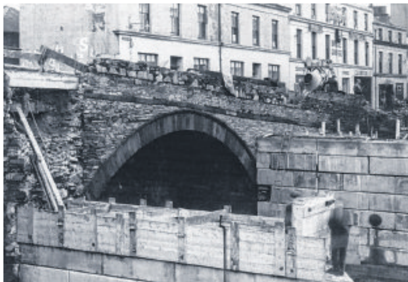
Constructing the central concrete pier for the replacement 'Stone Bridge' in 1936
