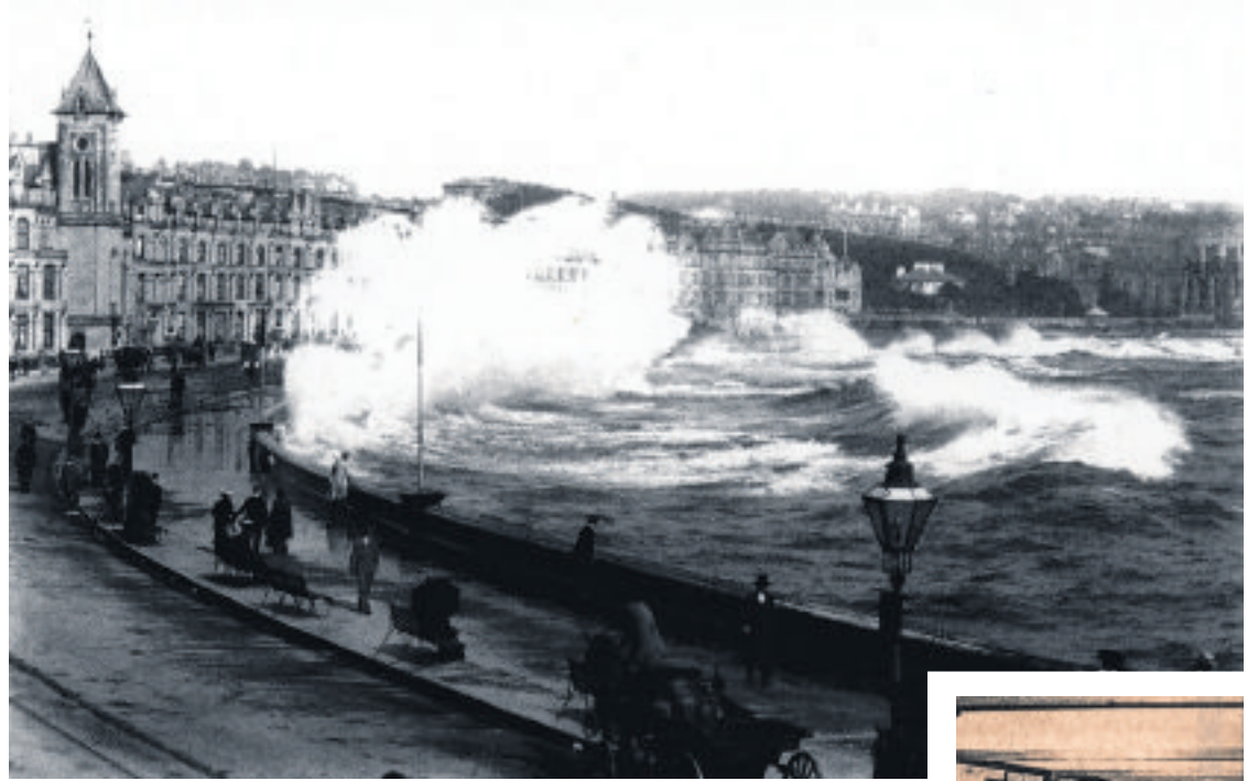
Power of the waves striking Douglas seafront prior to the promenade being widened
