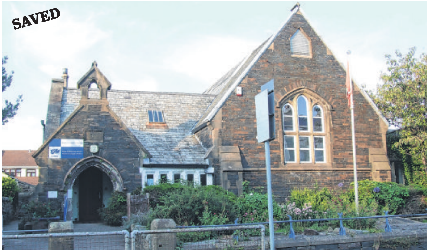
In his design for the Grammar School James Wild used the same gothic style that he used for the almshouses next door. They were built out of local stone with an imported stone (possibly York stone) for the window surrounds. Unfortunately somebody has decided in more recent times to paint over the natural stone of the window surrounds alongside the front door. Wild's most famous design was the Italianate hydraulic tower at Grimsby Docks based on Torre del Mangia in Siena
