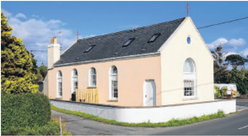
Ballakaneen, Andreas - there was a chapel on this site since at least 1782. The original chapel was replaced in 1863, and this building – the Sunday School – was added alongside in 1880. This became used as the chapel in 1982 when the chapel alongside was demolished. Now closed and converted to a dwelling
