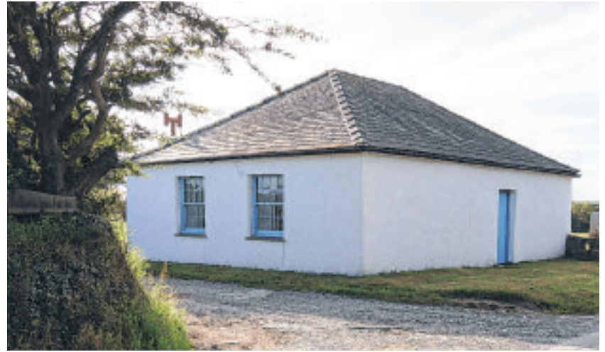
Former Leodest Chapel (in Andreas) which has since been sympathetically converted to a dwelling
