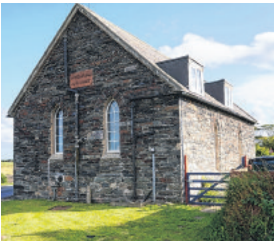
Glascoe Wesleyan Chapel in Bride, which was built in 1856 at a cost of £160. It closed as a chapel in 1965
