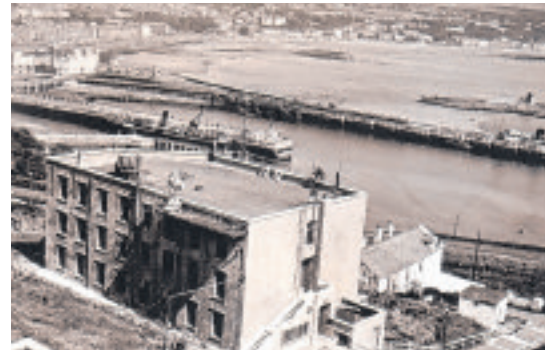
The HMS Valkyrie radar building is now the home of Manx Radio
