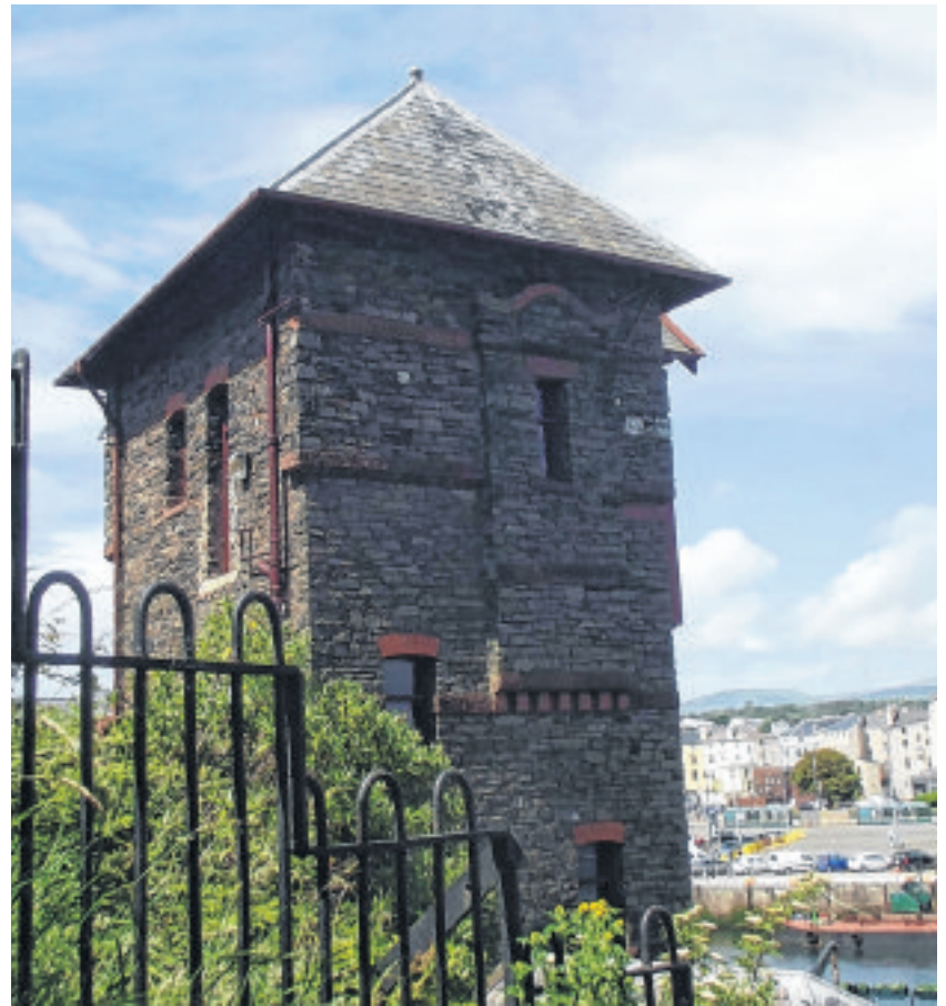
Former Douglas Harbour Swing Bridge control tower, which was built in 1895
