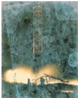
Warwick Tower on fire in 1906
