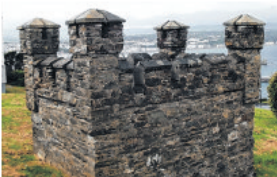
Castellated covered walls of Douglas Head
