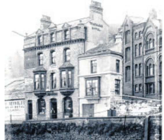
The Trafalgar in Douglas, formerly known as South Quay Tavern
