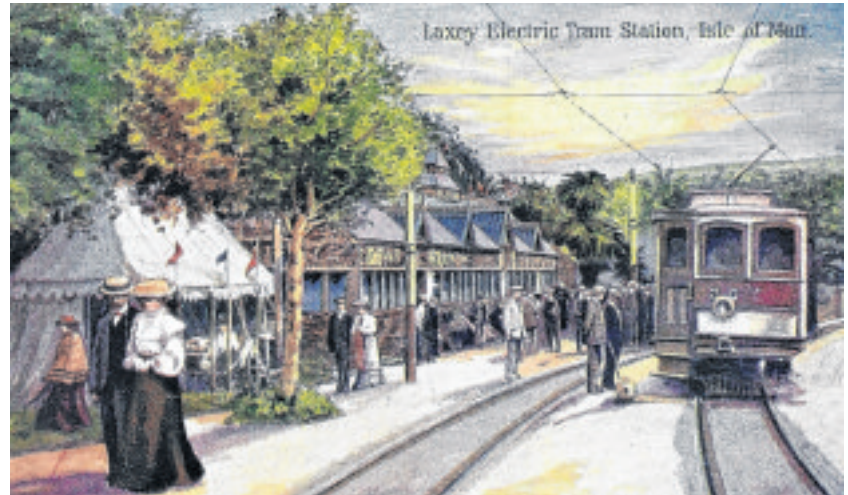
The refreshment rooms at Laxey station
