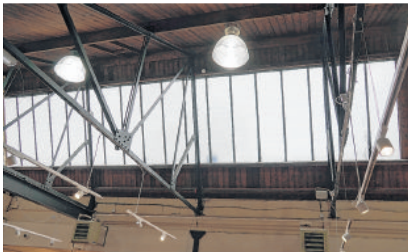
Roof-lit weaving and finishing shop at Tynwald Mills
