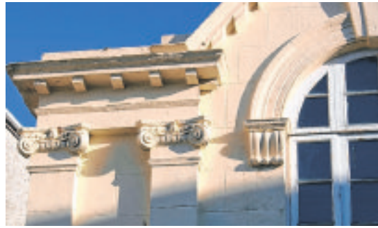
Carefully-detailed front elevation, with imitation-ashlar lines
