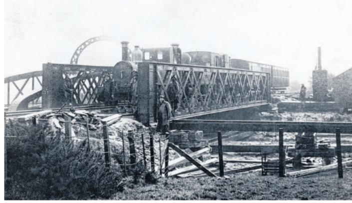
The new girder-framed replacement bridge at Ballakillinghan being tested in 1914, after being slid into place. Visible in the background is the 'handle' arch and sides of the 1878 'basket' bridge
