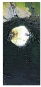
The bridge which carries the Milntown mill tail race under the Glen Auldyn road – only a couple of feet span but the bridge is effectively over 20 feet wide!
