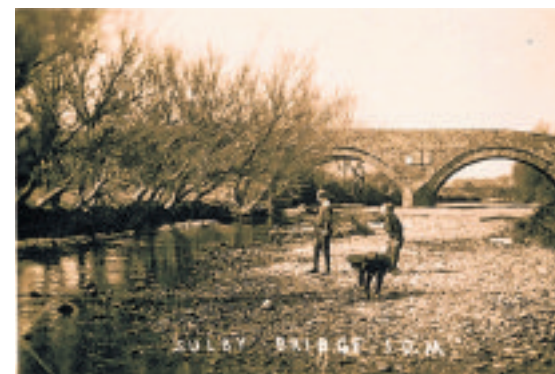
The previous stone Sulby Bridge, now supported on iron girders (photo: Manx Museum)
