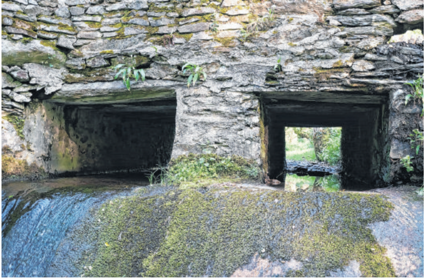
Narradale bridge with two 'slate'-slabbed square spans
