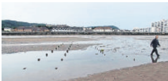
Four rows of landing stage supports
