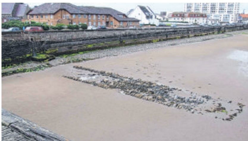
View of the Old Jetty from Queen's Pier c2016
