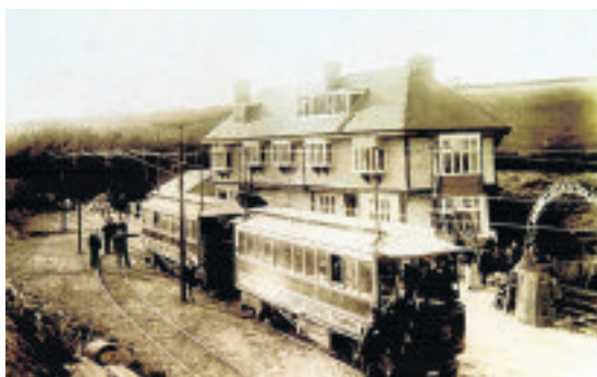
Tram number three prepares to return to Douglas. On the left contractor's materials and plant lie at the side of the line. On the roof of the hotel a cat ladder lies alongside the nearest dormer window. Beyond the hotel is a stable for three or four horses. When Richard Maltby Broadbent advertised for a manager he received 100 applications. He selected Mr Driver who had been the manager of the Injebreck Hotel and Pleasure Gardens at Baldwin
