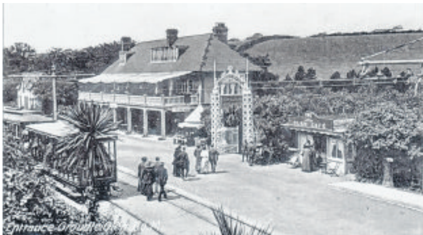
A view taken prior to the Great War as another load of passengers alight for a day at Grouldie. Baillie Scott's wooden veranda has been renewed in concrete but following the same design. The length has been extended to the full width of the frontage but the wooden balustrading has been reused. A canvas awning has been erected to shade those taking tea on the new balcony area opened up to the public. On the left of the hotel is a new two storey stable building which was timber framed then sheeted with expanded mesh and roughcast to match the hotel. On the right is a café erected in 1894 on stilts at the rear to provide a level floor. This building was erected as a temperance refreshment room utilising the landward pavilion from the Iron Pier at Broadway on Douglas Promenade which was being dismantled at that time. The first manager was Mr George Bowling
