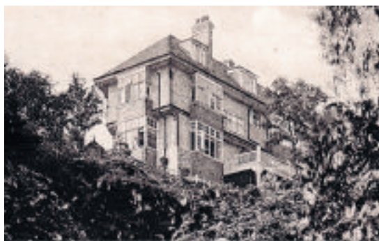
A rear view of the hotel taken from within the glen. Note the wooden balcony on the right which gave patrons the opportunity to look down into the glen. It was supported by wooden legs which were replaced in 1939 by a steel frame. In 1953 the lounge was extended out onto the balcony area. The basement walls are in exposed stonework whilst the walls between the different levels in the bay windows were hung with decorative shaped red clay tiles
