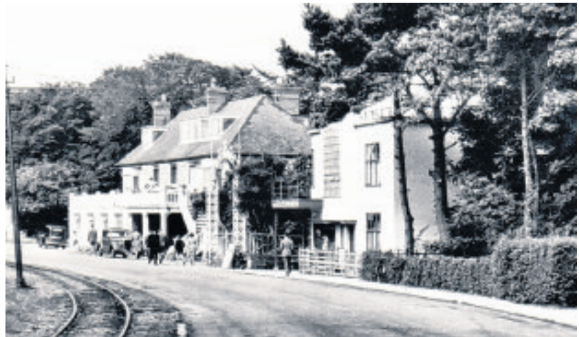
Probably taken in the years after the Second World War. Note the staircase created to provide direct access to the tea terrace. Four sections of the veranda have been filled in to provide additional room inside the building. To the right of the picture is Glenholme, erected to the designs of Lomas and Barrett in the 1930's as an example of 'Moderne' architecture. It provided living accommodation for the company manager but also contained a sweet and cigarette shop come ice-cream and pop café at ground floor and first floor level with its own balcony. Beneath the dwelling were spacious public toilets for the patrons of the glen
