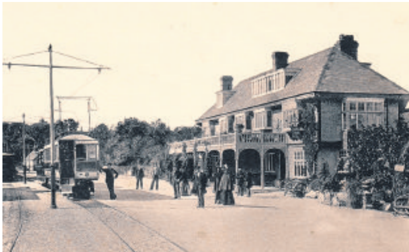
A picture taken post 1894 when not only has the veranda been built but there are creepers growing up the legs. A garden has been created at the entrance to the glen and off to the left a large waiting area and booking office have been built. These stand to this day having been renovated in 1993 under the directions of Maurice Faragher from the MER. Note the electrical connectors on the tram being the same as to be used on the Snaefell Mountain Railway.
