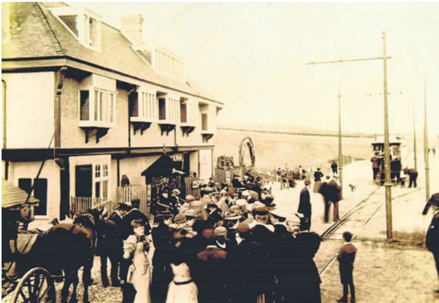
An extremely rare picture taken on September 7 1893 when the first electric trams ran between Derby Castle and Groudle on a single track with a passing loop on the right of the picture. Baillie Scott's Groudle Glen Hotel looks strange without the intended veranda which was constructed before the 1894 season. The flat roofed dormer windows and the small bay windows suspended from the overhang above were used for the first time on this building. They later became iconic of Scott's work. Also visible are the carved wooden corbels set diagonally on each corner. Note the complete lack of trees in the glen on either side of the valley
