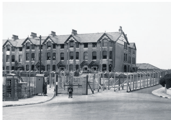
A K6 kiosk outside the internment camp at Port Jack Glen
