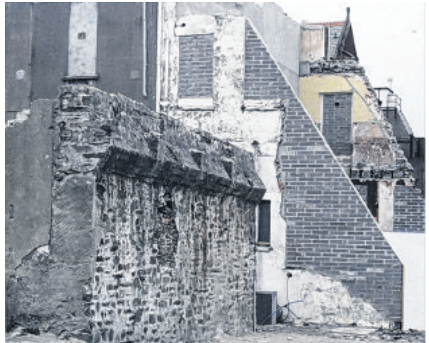
Douglas Sea Wall (Villiers site)
