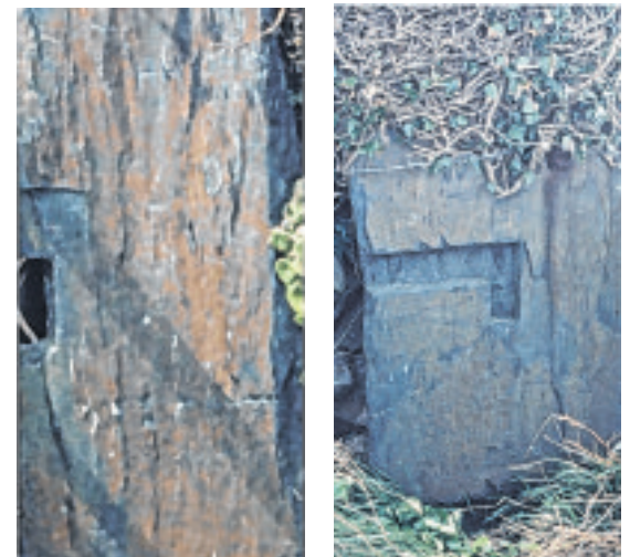
Pair of gateposts with holes and slots for wooden bars (1994)
