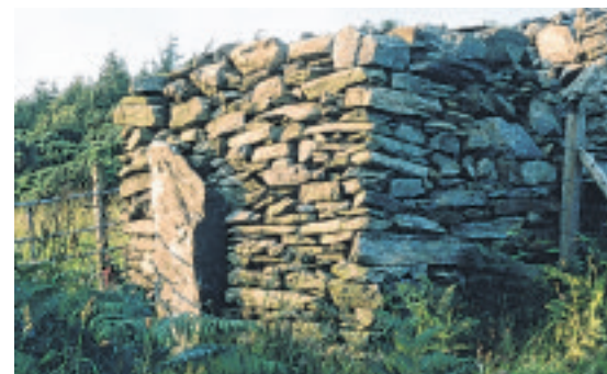
Grand field walls in the Laxey valley (1997)
