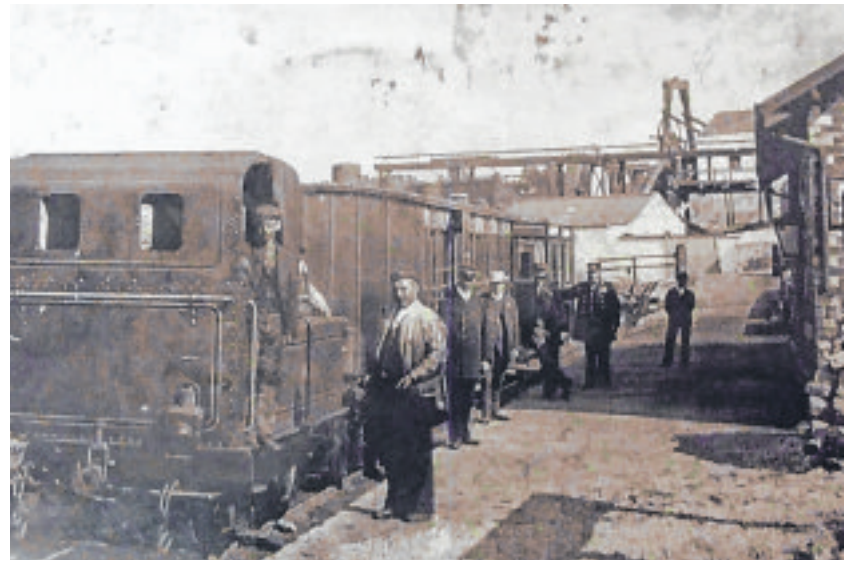
A branch line train at Foxdale station, ready to return to the junction with the Peel and Ramsey lines at St John's. The viaduct and clock tower are in the background (Picture courtesy of the iMuseum)
