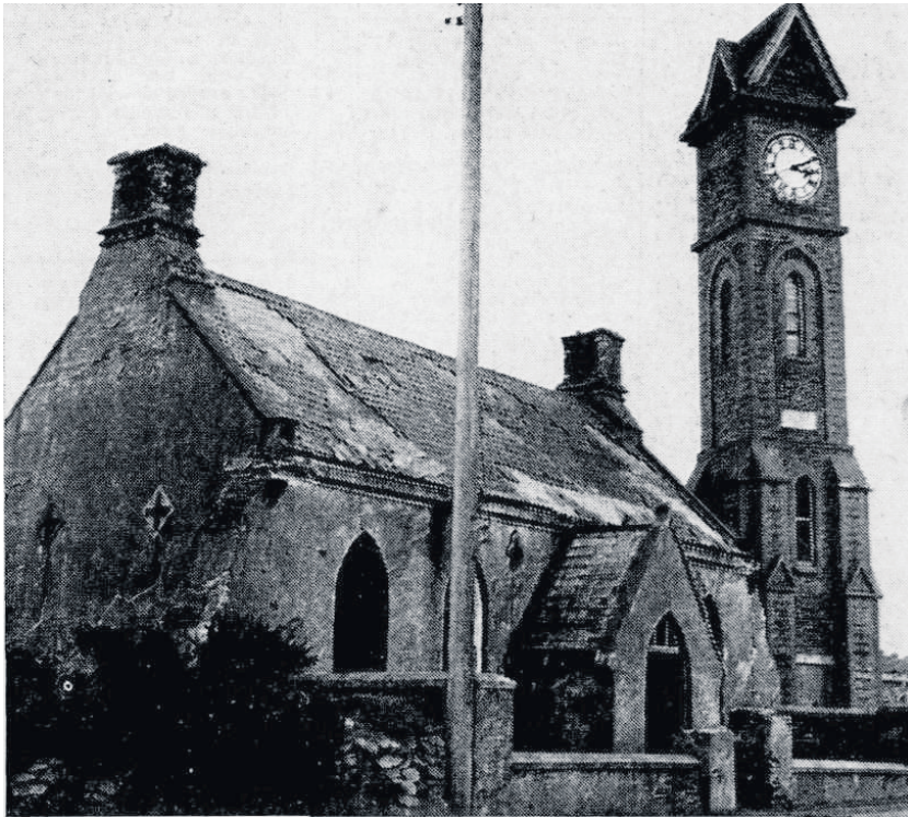
Foxdale working men's institute and clock tower
