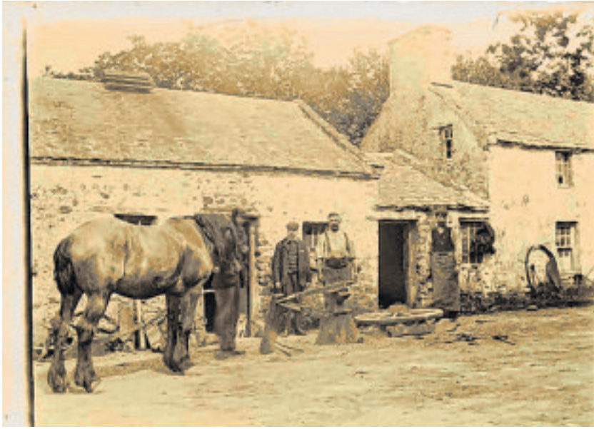
Undated image of a busy working day with a wheel ready for hooping. Smiths preferred to shoe horses indoors as it made them easier to control. Horse shoeing was prioritised over other work (Picture courtesy of MNH)
