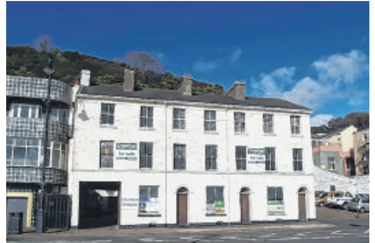
The frontage of Tramway Terrace
