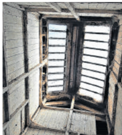
Looking up at the stables' clerestory roof
