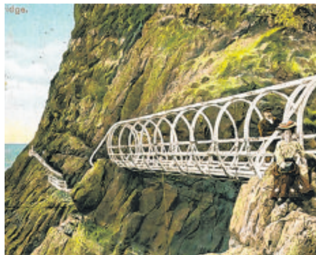
The impressive Tubular Bridge was made up of circular steel rings
