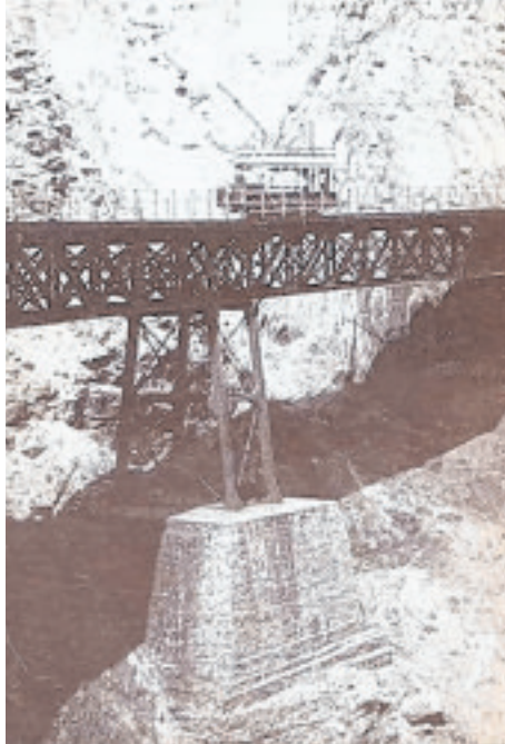
A tram using the viaduct
