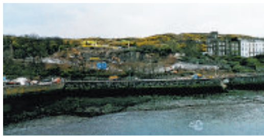
The Fort Anne site is cleared before being rebuilt in 1997
