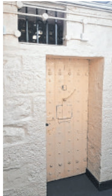
Cell door and double-barred ventilator/window
