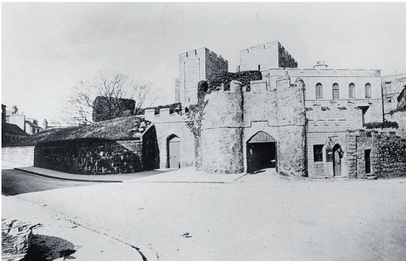
Original Police Station (to the right of the Castle gates) and construction starting on the new Baillie Scott station – bottom left of picture (Manx Museum)
