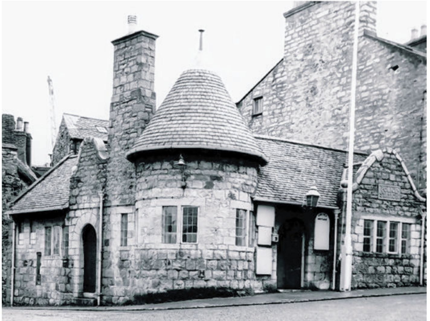
Baillie Scott's police station – distinctive conical roofed tower and shaped gable that he used in his competition design for 'House for an art lover'
