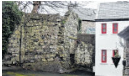
Part of the boundary wall
