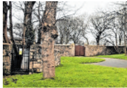
Part of walled garden and former farm buildings
