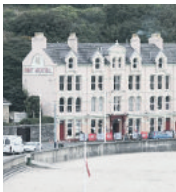
The Bay Hotel, Port Erin, renovated by Martin Brunnschweiler, is now a successful pub
