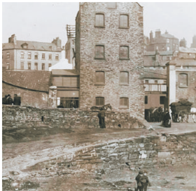
Clinch's Brewery in the early years of the twentieth century. Fresh water for the brewing process was obtained on the Artesian Well principle. The original Georgian brewery buildings were in the yard at the rear nestling under the embankment supporting Big Well Street, later to become Lord Street.
