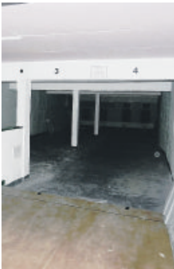
An interior view of part of the building
